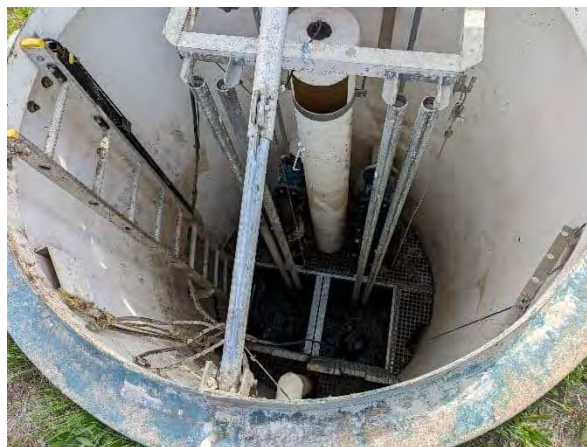
Figure 2-3 Collis LS Internals
