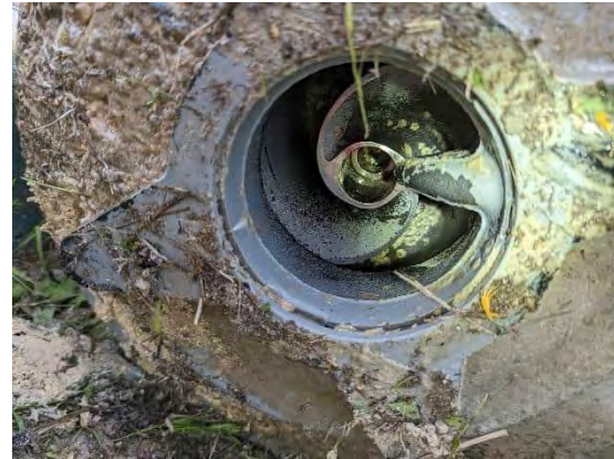
Figure 3-4 Pump 2 Impeller
